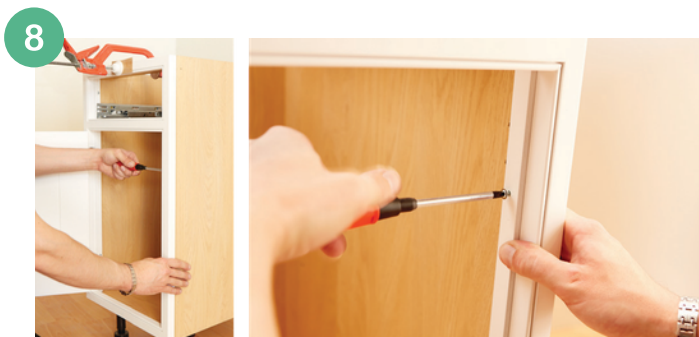
8 Using a fixed handle screwdriver, screw the fixing bars with the 3.5x30mm flat head screws provided (this avoids over tightening and will not put strain on the frame).
